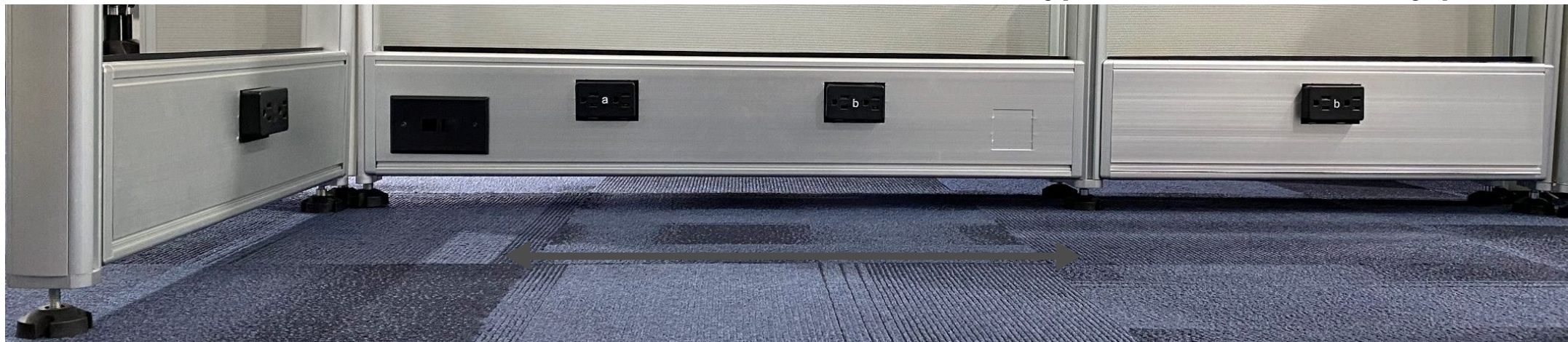
Typical Electrical Raceway (covered)
